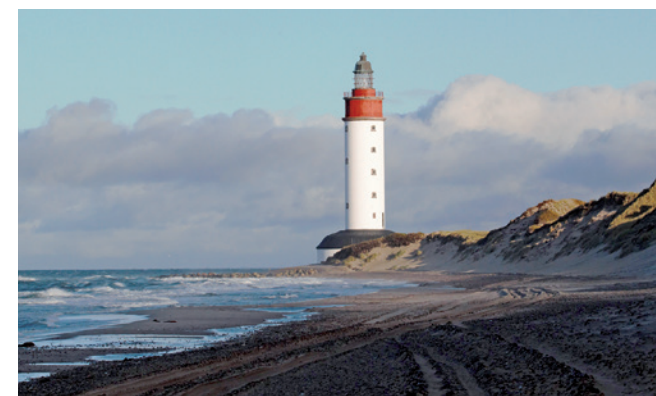
Anholt Lighthouse – built 1785-1788 and heightened 1881.
